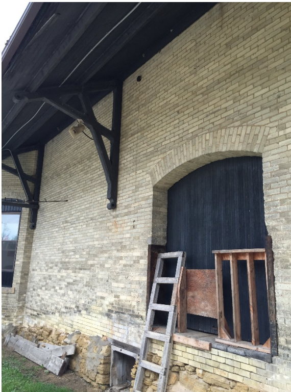
Original Pulley Door – West Façade
