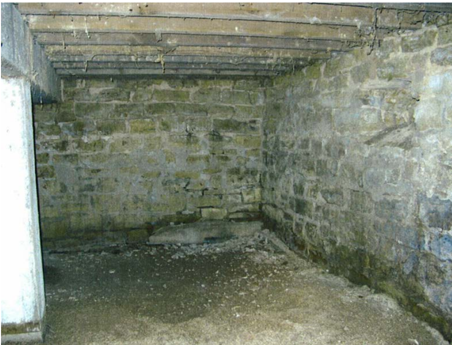
Basement crawl space with limestone foundation
