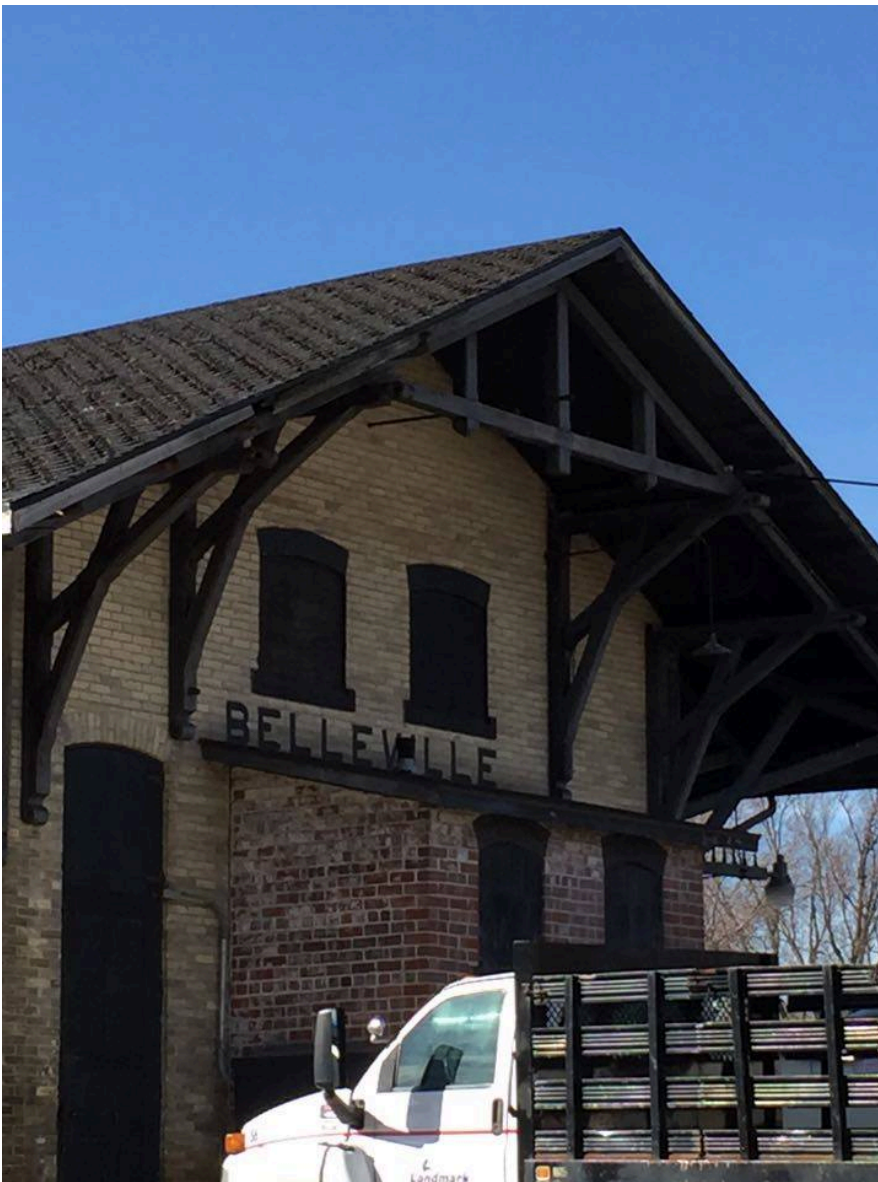
North Facade – Gable Detail
