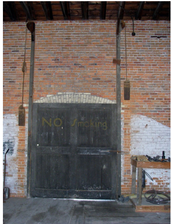
Interior at Pulley Door
