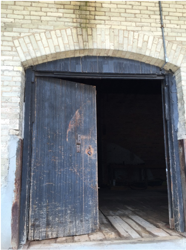
Original Freight Door
