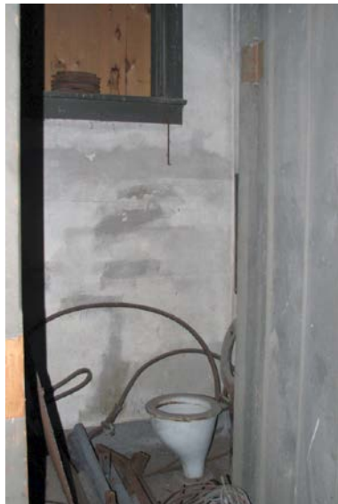
Existing Water Closet
