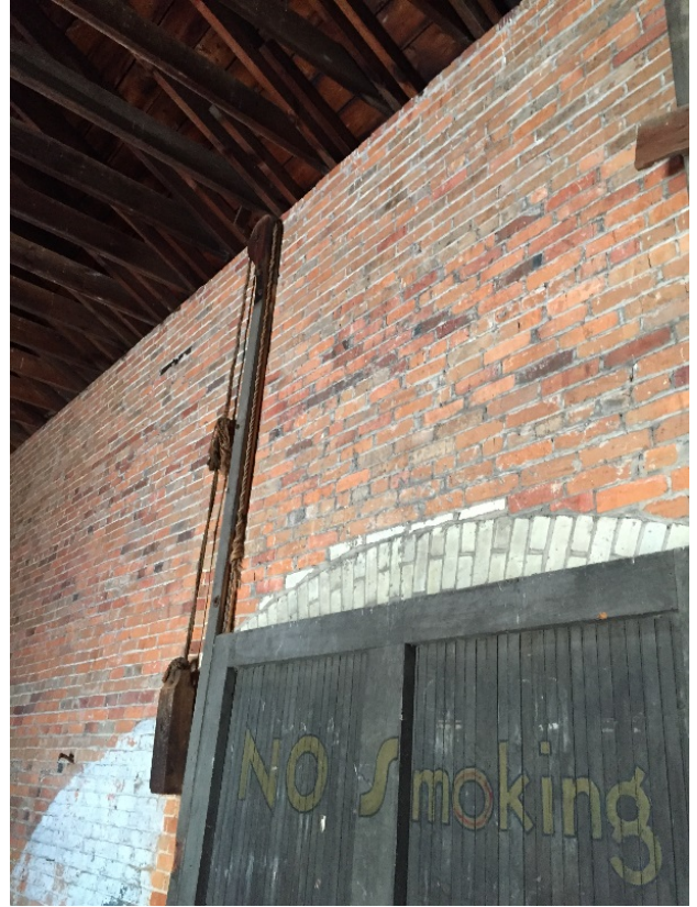
Freight Area with Pulley Door
