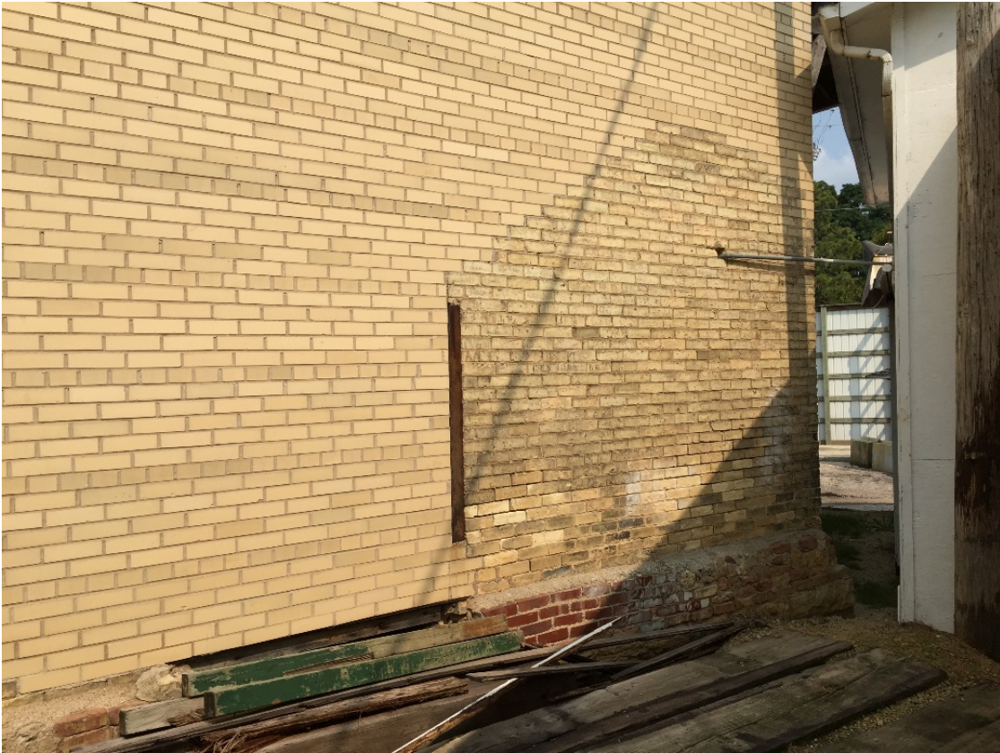
South wall – Non-historic Brick Condition, Exterior
