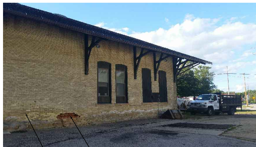
AREA # 1- BRICK / STONE DETERIORATION @ BASE
