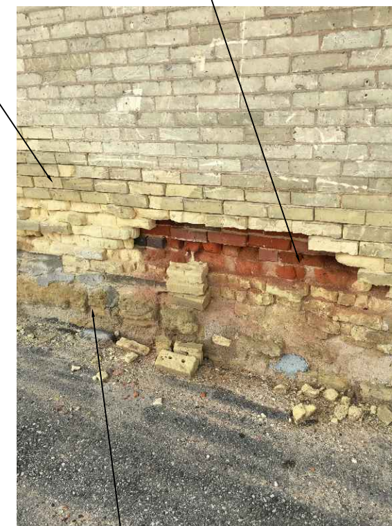
AREA # 1- BRICK / STONE DETERIORATION @ BASE
